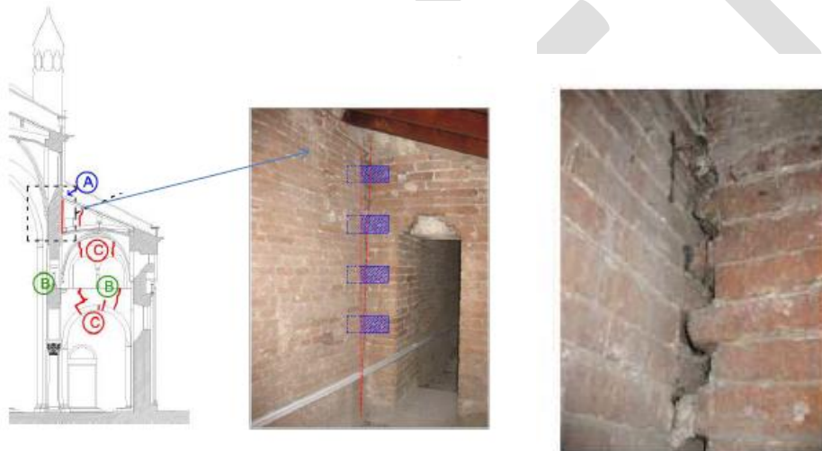
Figure 75: Connection of the orthogonal walls
