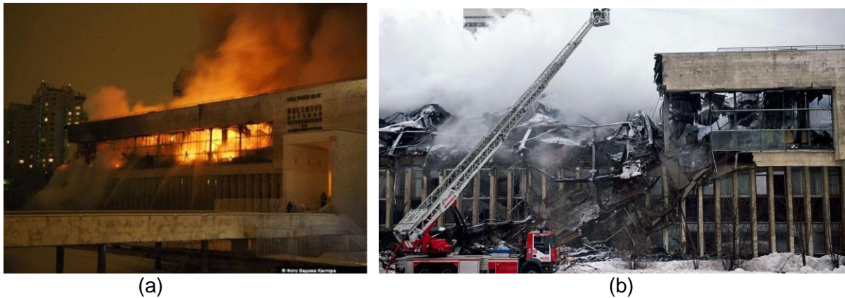
Figure 6: Case of the Science Academy Library in Moscow. Fire development exterior view (a); after-fire exterior view (b).
