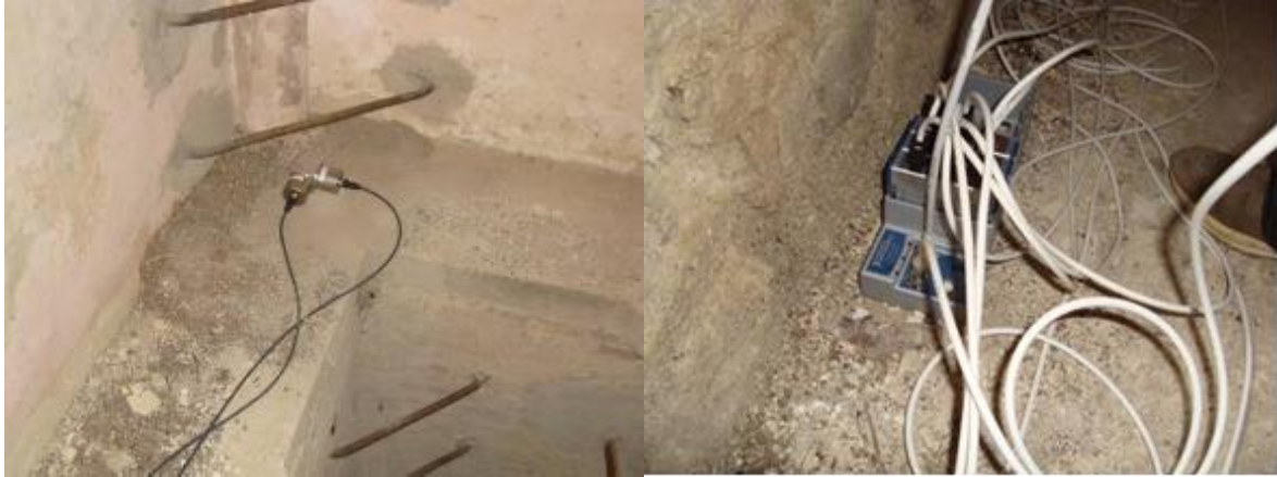
FIGURE 33 PIEZOELECTRIC ACCELEROMETERS POSITIONED AT THE SOUTH-WEST CORNER OF THE TOWER AT 12.5M
