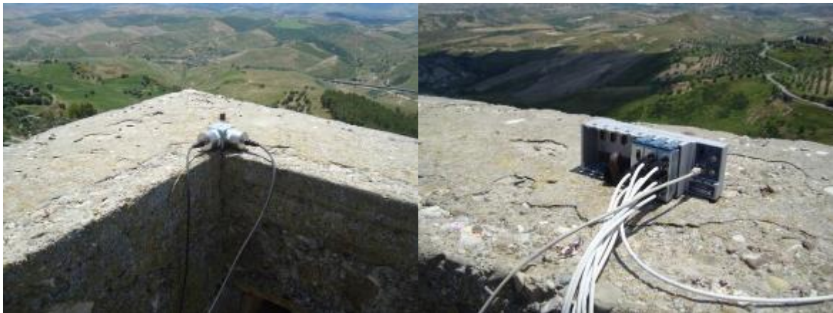
FIGURE 35 PIEZOELECTRIC ACCELEROMETERS POSITIONED AT THE SOUTH-EAST CORNER OF THE TOWER ROOF AT A QUOTE OF 21 M
