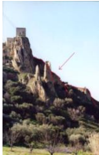
FIGURE 8 – DETACHMENT SURFACES OF COLLAPSES ALONG THE CONGLOMERATE WALLS OF THE NORTH-EASTERN SLOPE.
