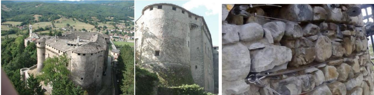
Figure 1.4.10: Application of Reticulatus technique to the Castle of Compiano [22]
