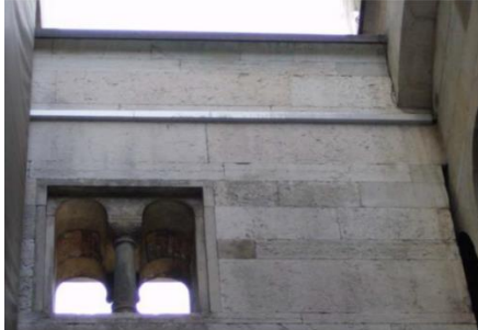
Figure 2.2.39: Deformer installed on the buttress of the Cathedral (D1)
