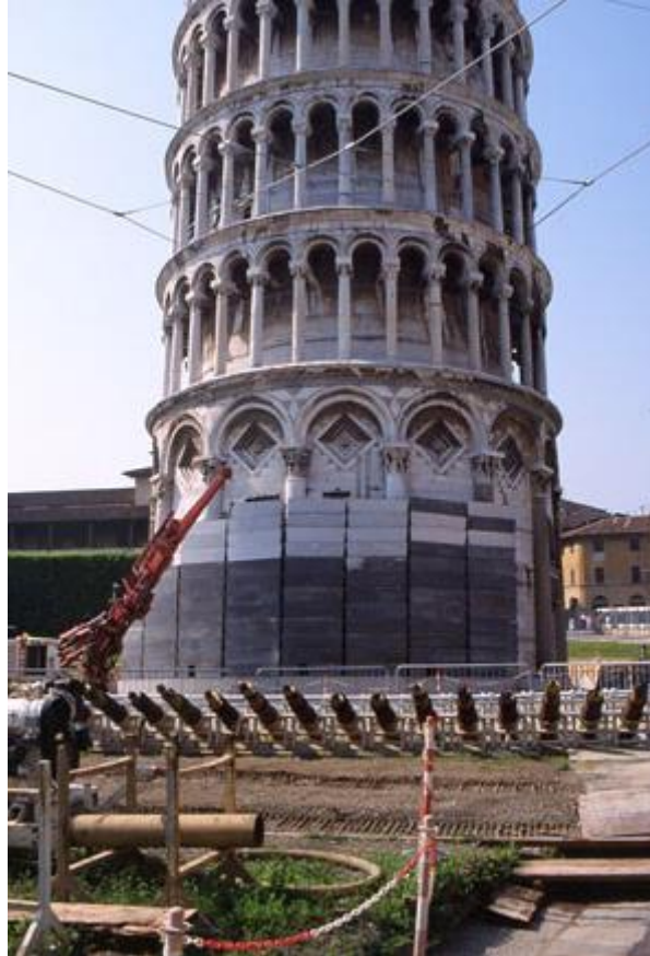
Figure 1.4.6: Under-excavation work and tensioned cables
