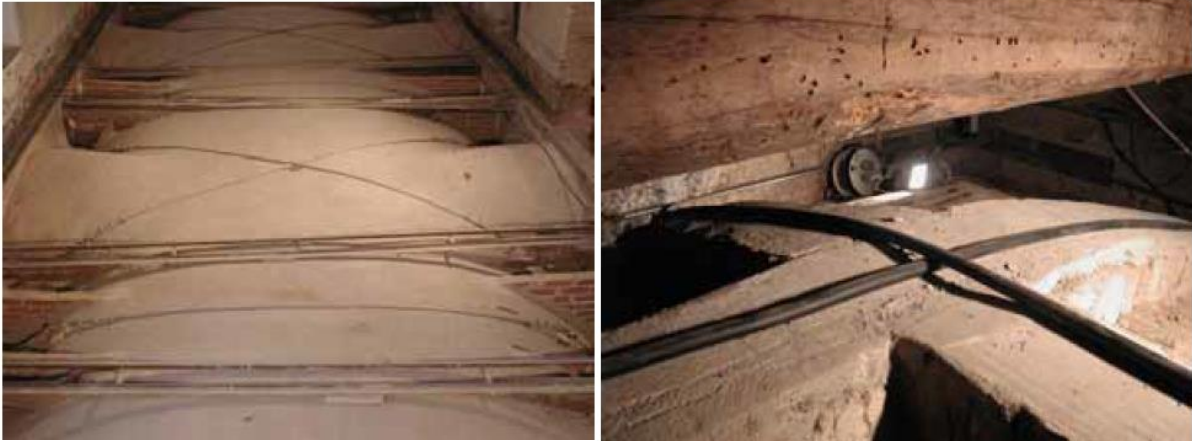
Figure 1.4.11: Application of “reinforced arch method” to the vaults of Casa Giacobbe (Milan) and Manta Castle (Cuneo) [26].
