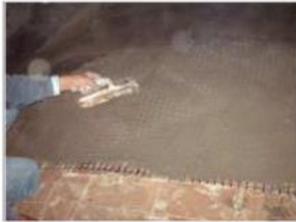
Interventions for strengthening the vaults: a) extension of the "frenelli"; b) layer of lime added with eco-pozzolana and reinforced with carbon-fiber mesh
