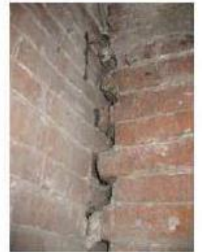
Connection of the orthogonal walls
