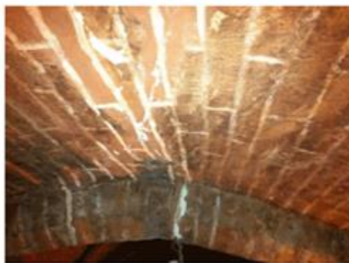
Figure 71: Consolidation of the decorated plaster with using compatible pigments
